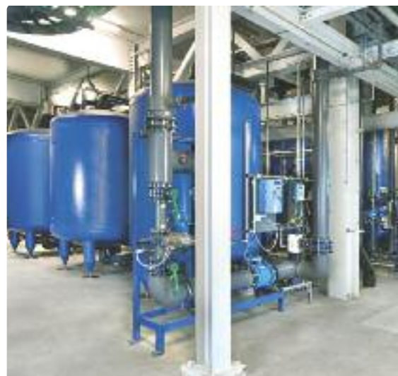
A 200m 3 /hr water softening plant and blending unit with hardness monitoring in a modern Dutch brewery.
