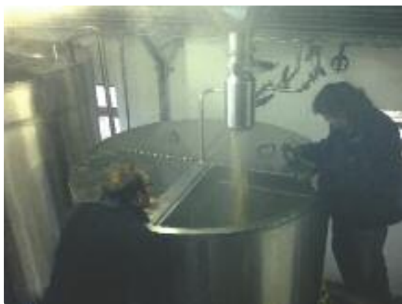
A 200m 3 /hr water softening plant and blending unit with hardness monitoring in a modern Dutch brewery.
