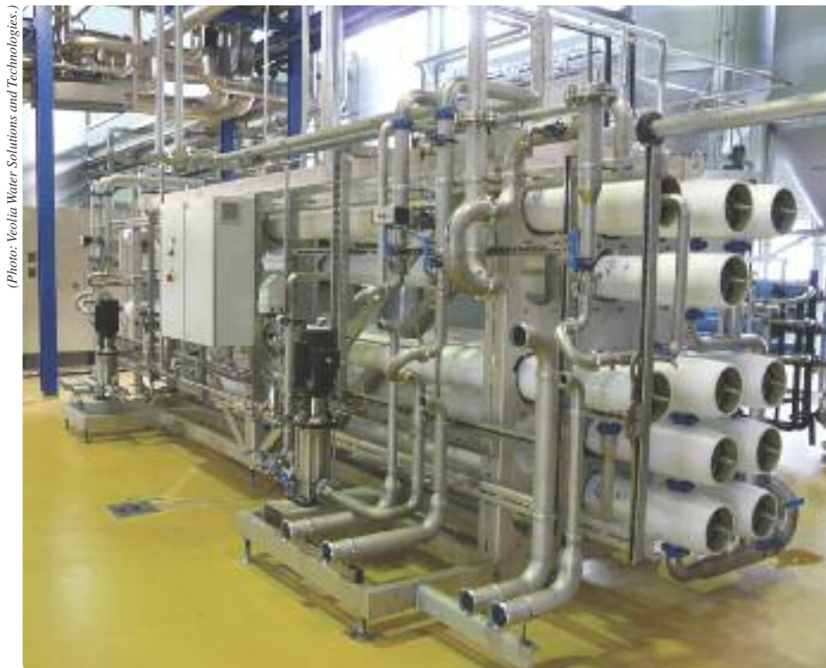
A 93% recovery, 60m 3 /hr reverse osmosis plant in a modern German brewery.
