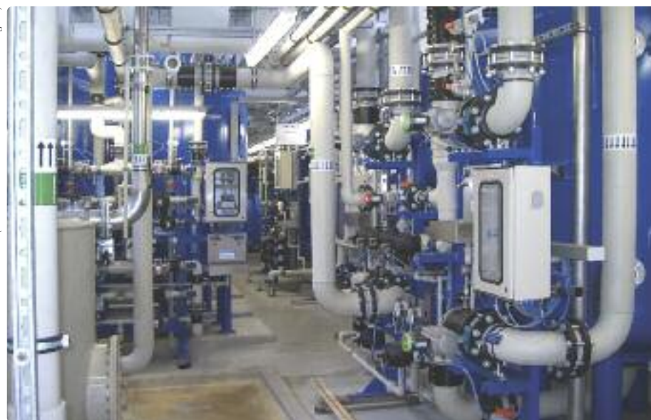
Cation and Anion demineralisation equipment in a modern German brewery.
