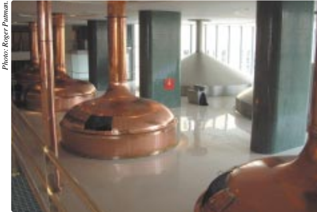
Figure 2: Pilsner Urquell brewhouse (2004). Note the copper clad vessels with one of two 10m lauter tuns in the back ground. Over 100,000 visitors a year inspect this view from an elevated walkway.
